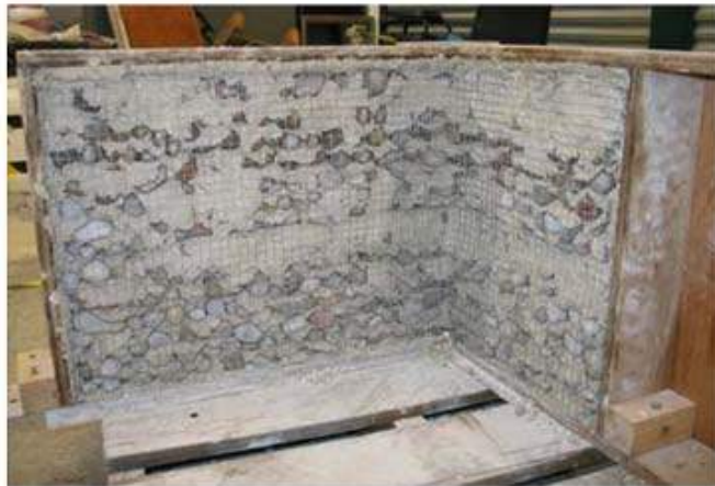
(a) Steel cage
