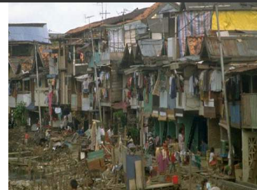
Seismically non-resilient residential construction
